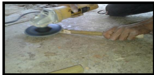
Fig8(a) Preparation of Bamboo panel
