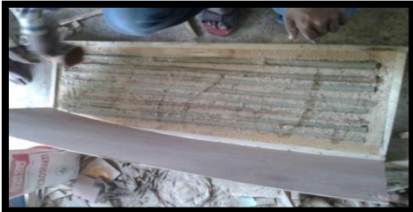
Fig8(e) Preparation of Bamboo panel
