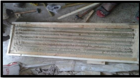
Fig8(d) Preparation of Bamboo panel
