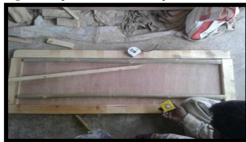
Fig8(b) Preparation of Bamboo panel
